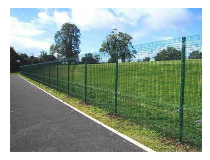
Fig 72. Illustrative example of 2.4m high paladin security fence
